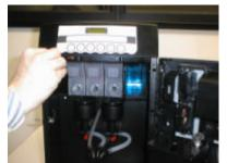
Then **insert the safety key** into the safety switch as shown in the picture.
